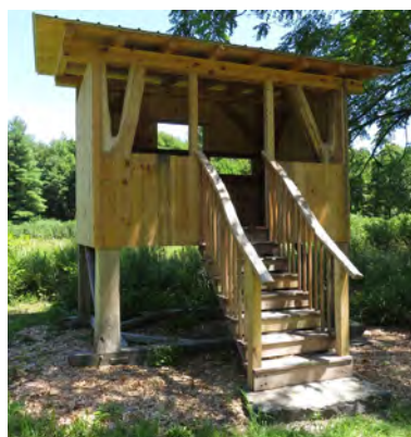
The finished blind overlooks one of Northampton's most extensive marshes
