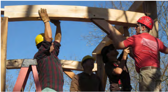
Fitting an arched beam into the blind's timber framework
