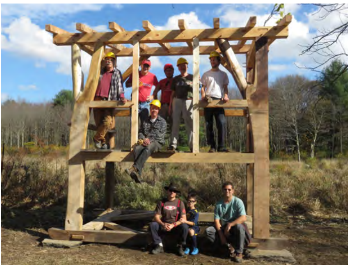
The blind's frame was fitted together with no metal hardware
