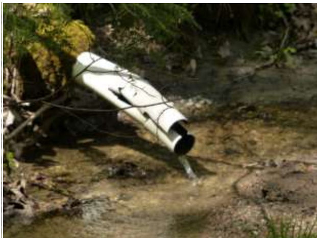
A pipe from a nearby property owner's sump pump extends to the brook.
