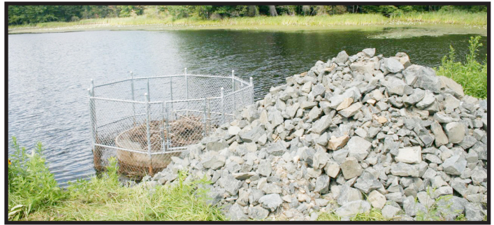
A big pile of rock was delivered to the edge of the dam, ready to be moved by hand to the fence around the drain. (Bob Zimmermann)
