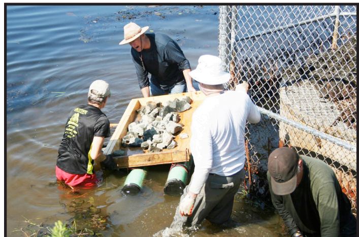
Innovation was required for the task of moving 10 tons of rock. Volunteers built a wooden chute to get the rocks to the water's edge and a float to move them around the perimeter of the fence. (Bob Zimmermann)
