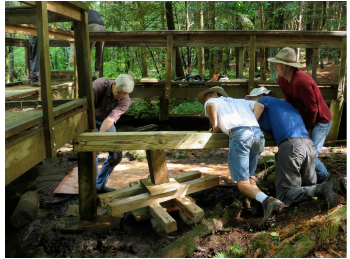
Volunteers raise the bridge to level the structure, which was listing badly. (Bob Zimmermann)
