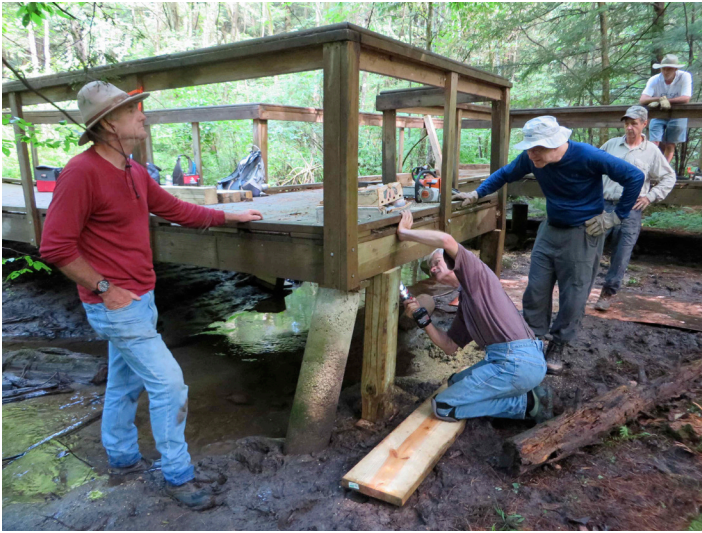
Bob Rundquist does the drill work while his co-workers, Steve Harding, Lewis Popper, Jim Reis and Jon Sass, look on. The bridge repair, while no small engineering feat, is not a permanent fix. (Bob Zimmermann)
