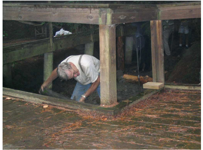
Bob Rundquist works on shoring up BOB. Photo by Bob Zimmermann.
